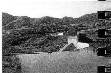
Railroad Canyon Lake Dam, built in 1928, created Canyon Lake, a water supply reservoir.
