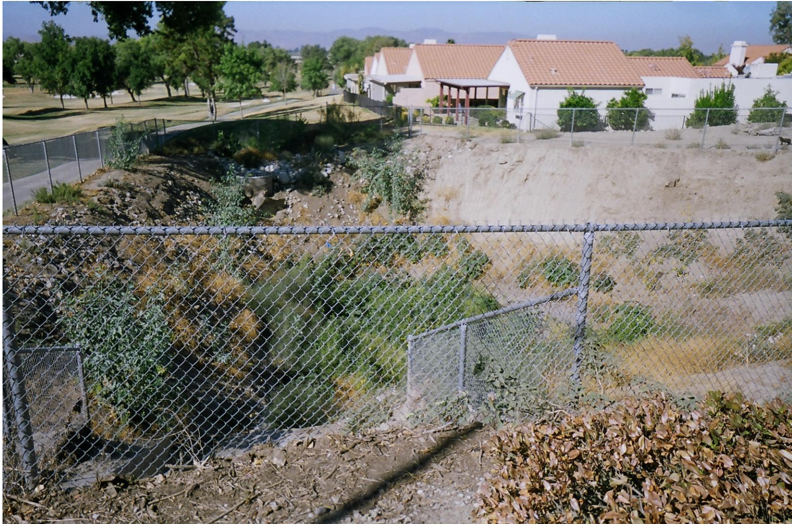
FIGURE 3-9 DETENTION BASIN DOWNSTREAM OF BOX CULVERT ON THE PROJECT SITE
