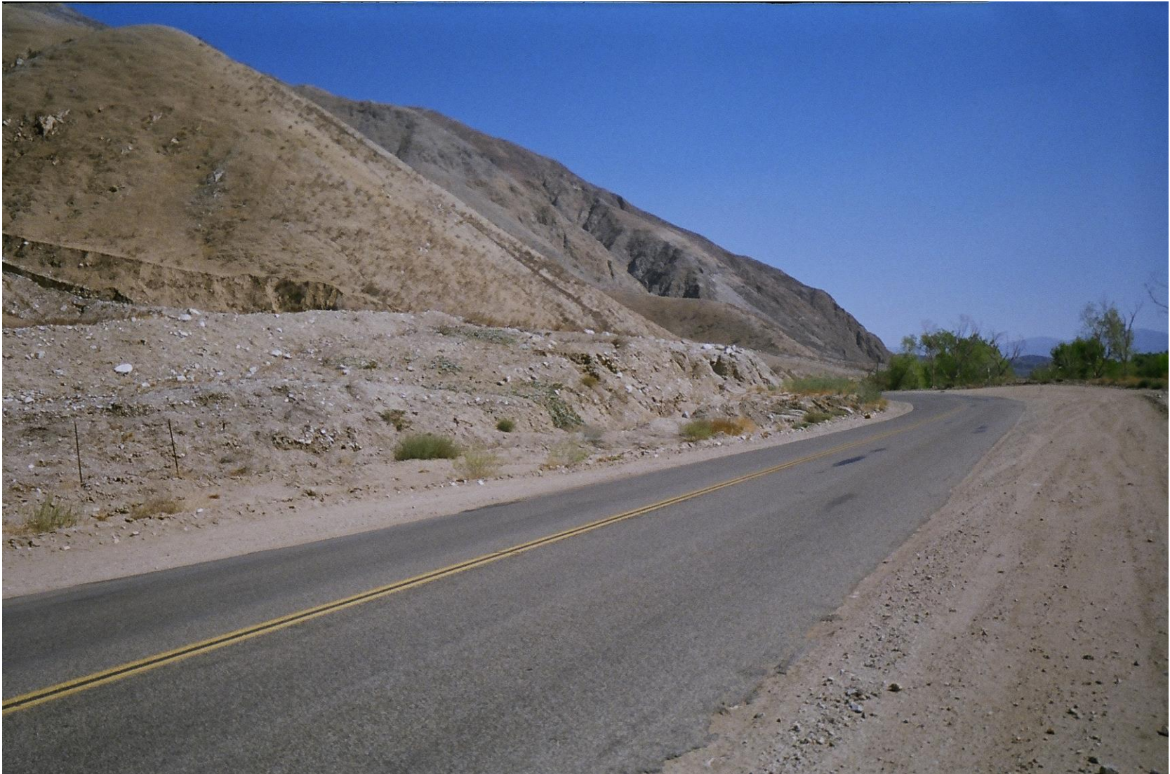
FIGURE 3-10 EDGE OF ALLUVIAL FAN NEAR SOBOBA ROAD
